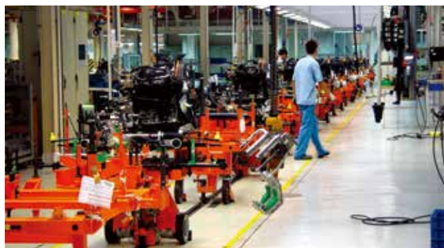
图3：LD母线槽系统作为理想的大电流输配电设备被广泛应用在工矿企业，例如图中应用在上海大众汽车装配流水线。 Figure 3: LD system is the ideal busbar for heavy current power distribution and transportation. It is mainly applied in industrial and mineral workshop, etc. e.g. common in applying for auto industry, Shanghai Volkswagen.
